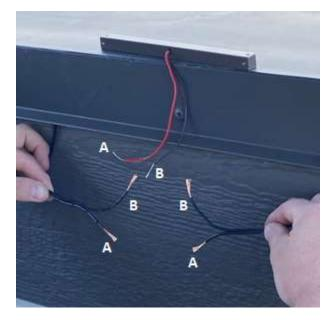
See example above, the main line pictured has a plain black wire & a black wire with a white line. These 2 wires will be reattached along with the red wire from the fixture. Make note to install each fixture the same. (i.e. if you install the red wire to the black/white main wire, do the same for each fixture). In this example, the wires labeled A will be attached to each other, and wires labeled B will be attached to each other. Use silicone filled wire nuts & wrap with electrical tape.
